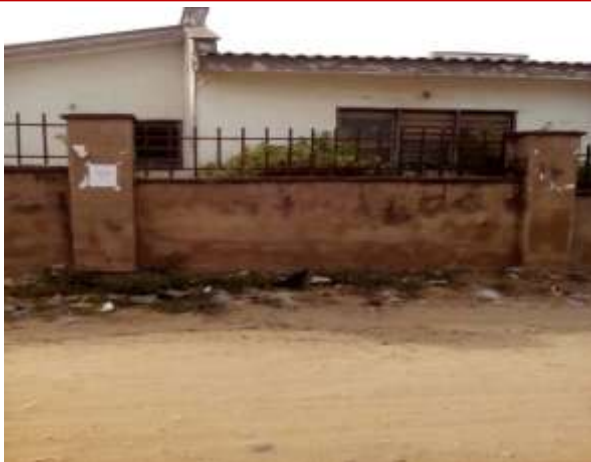
Some Building Units at the Shagari Low-Cost Estate, Lokoja
